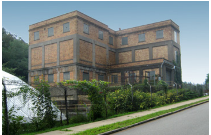
Hays Mine Station Chemical Treatment Plant
