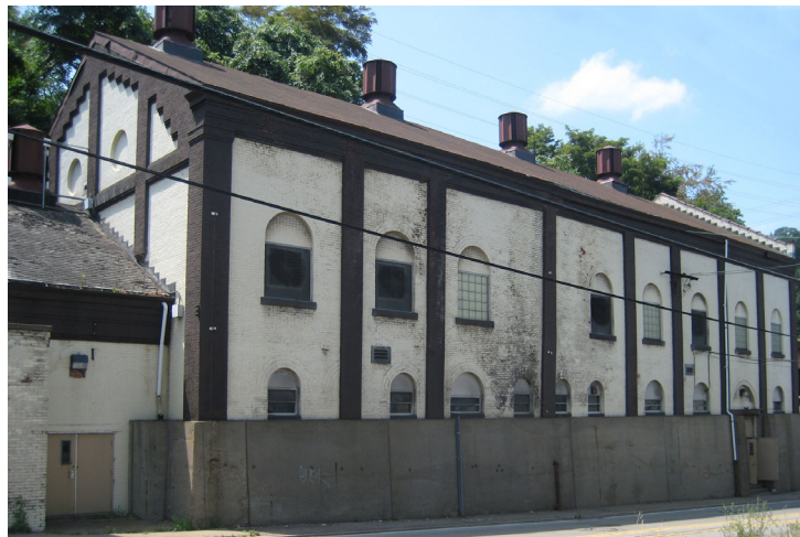
Becks Run Water Pumping Station
