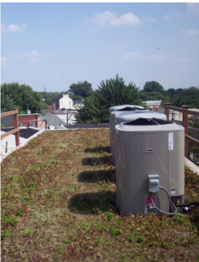
Green roof at 3933 Lancaster Avenue
